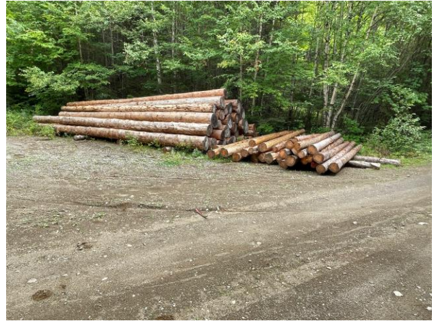
Logs on Site Ready for Construction
